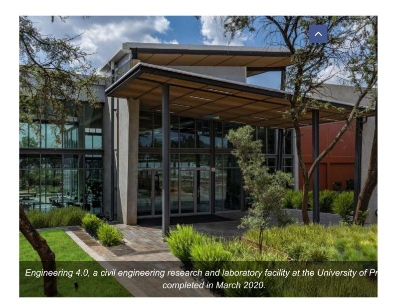
The glass foyer frame is made up of H- and I-beams creating a linear and radial grid that intersects through a forest area, creating a relationship between the interior space and surrounding environment. H-beams emphasise the rotation of each column along the radia walkway, while horizontal I-beams create continuity between the vertical and horizontal ele and connections between the two.
