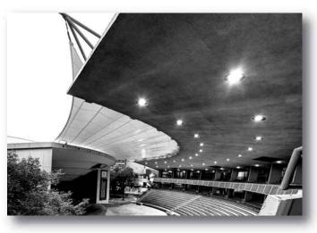
The amphitheatre accommodates a 3 000 seated audience in a two-tiered semi-circular roofed concrete structure, which is placed 14m detached from the external stage area on a radial pattern.
